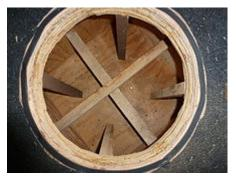
Heavily braced and built subwoofer enclosure
